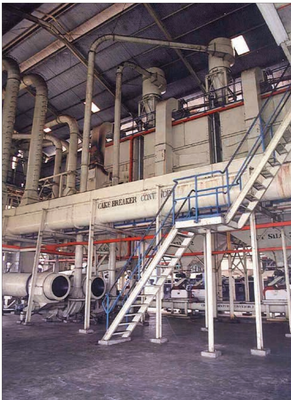
Cake Breaker Conveyor
