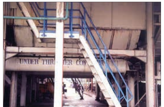
Under Thresher Conveyor
