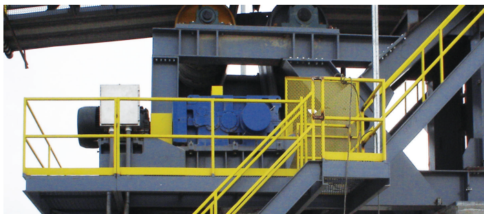
Paramax conveyor drive
