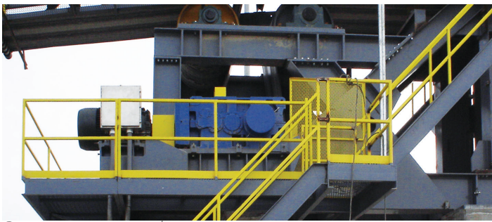
Paramax conveyor drive
