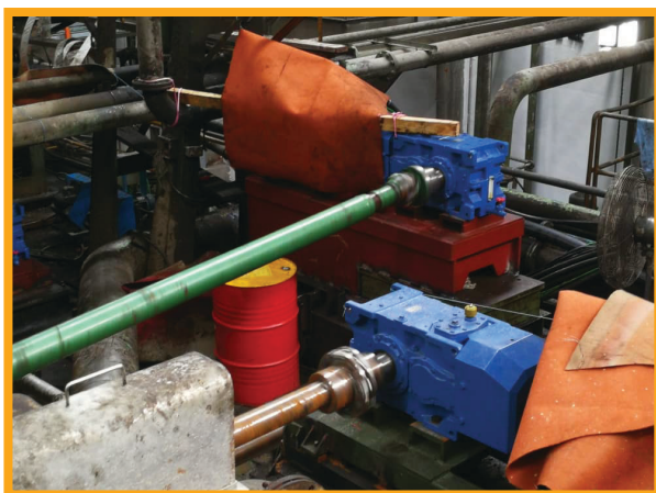
Replacement of our Paramax Right Angle, equipped with Double Reduction with fan, <60C max operating temperature with new baseplate.
