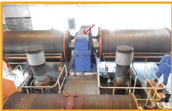
Replaced by Sumitomo YHD150P3A-BB-40.017 drop-in gearbox with 100% matching mounting dimension and excellent on-site support
